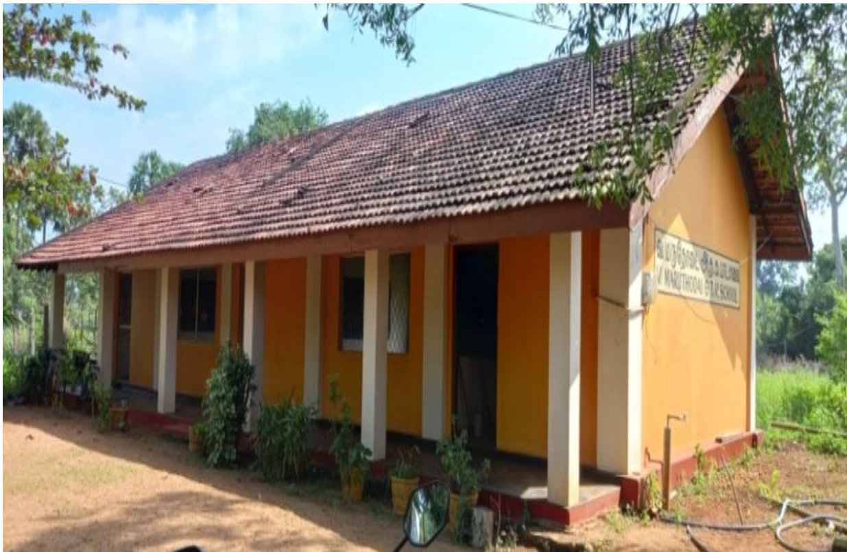
Figure 10 Repairs to class room Building at V/Maruthodai GTMS
