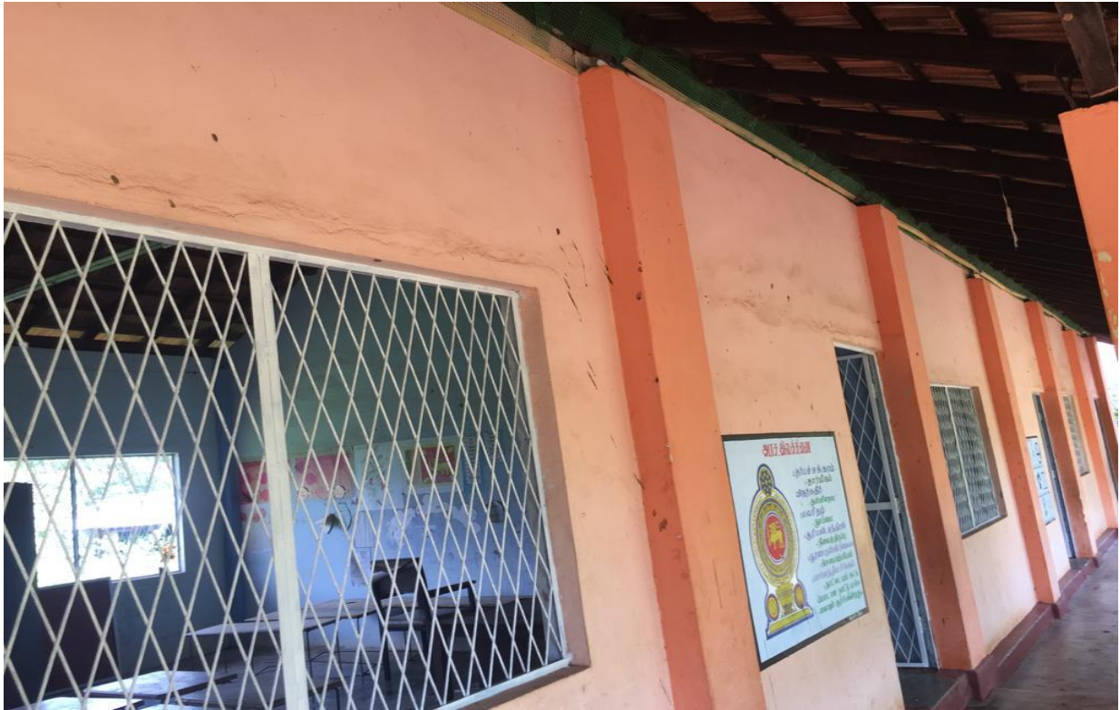
Figure 9 Repairs to class room Building at V/ Palayawady GTMS
