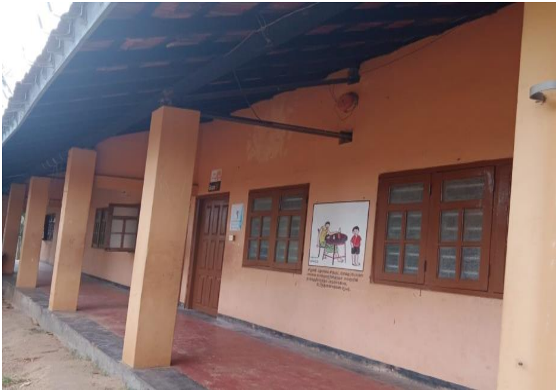
Figure 13 Repairs to class room Building at V/Kidachchuri Karuveppankulam GTMS.
