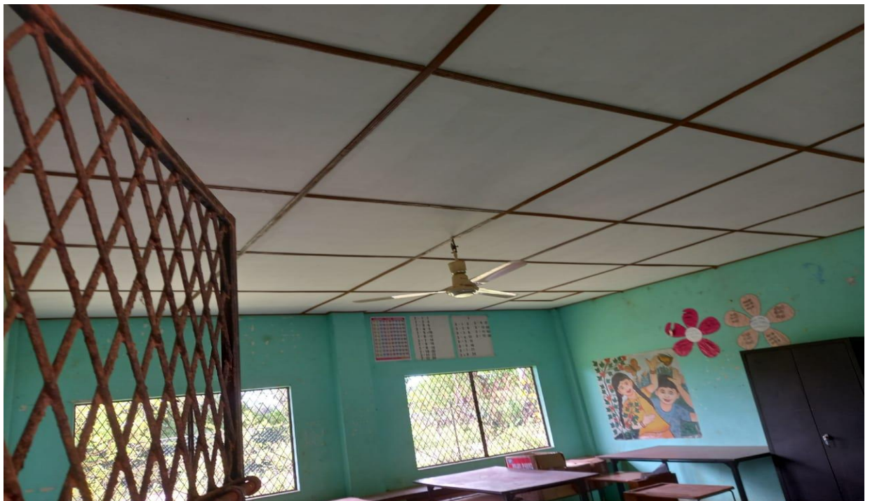
Figure 6 Repairs to class room Building at V/Marukkarampalai GTMS
