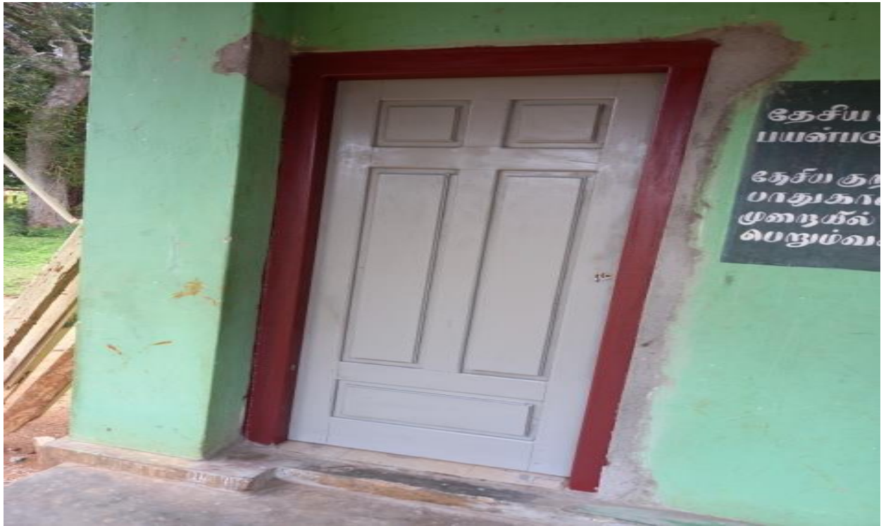
Figure 5 Repairs to class room Building at V/Kaddayarkulam Thiruvalluvar Vid.
