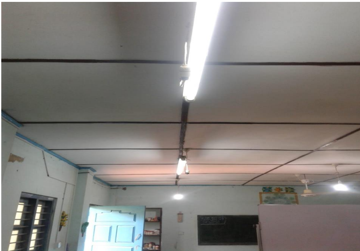
Figure 12 Repairs of science lab building V/ Poompugar Kannaki vid
