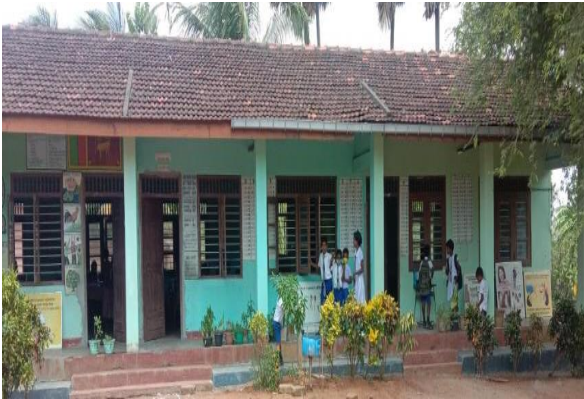
Figure 11 Repairs to class room Building at V/ Mathiyamadu Viveganantha Vid
