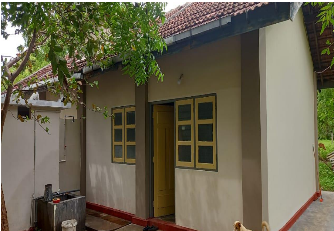
Figure 14 Repairs of teachers' quarter at V/Kalmadu M.V
