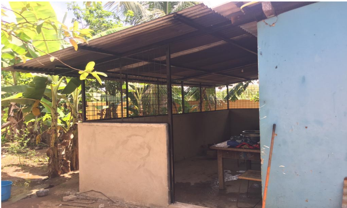
Figure 8 Repairs to class room Building at V/Senaippulavu Umaiya Vidyalayam
