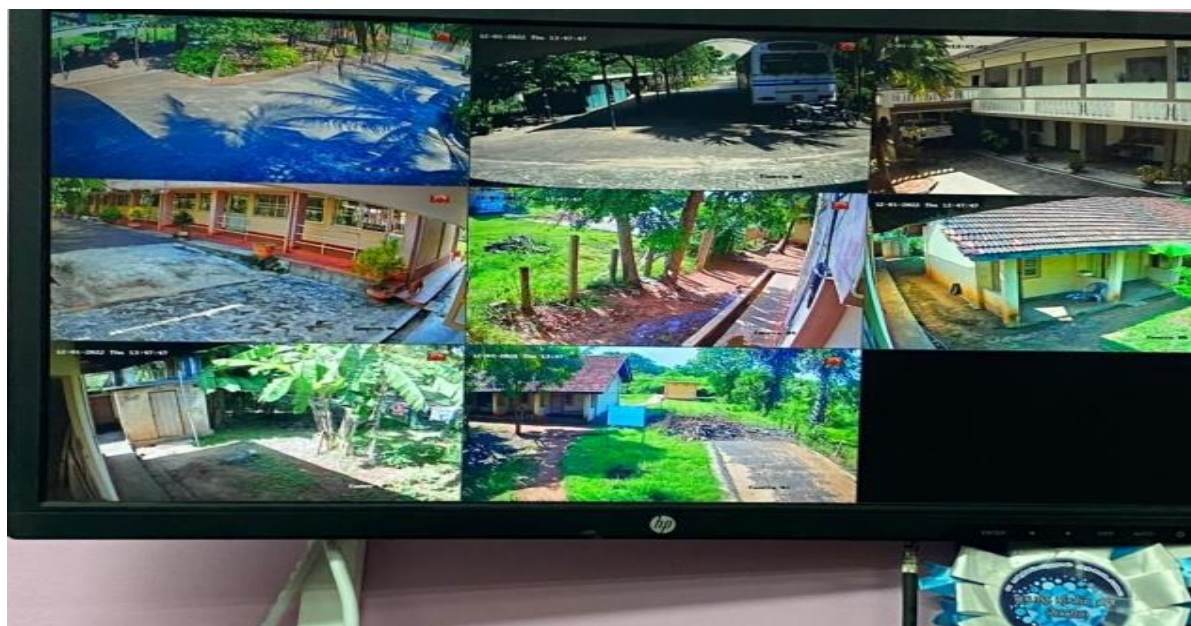
Figure 17 Installation of CCTV Camera at Zonal Education Office, Vavuniya North
