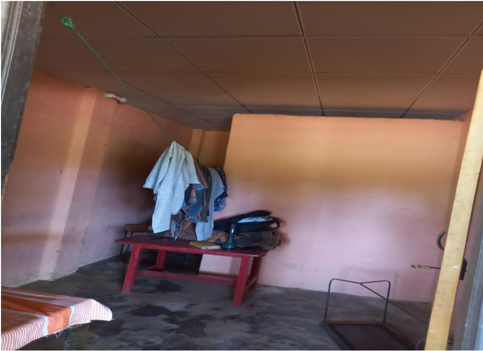
Figure 22 Renovation of Teachers' Quarters at V/ Kovilkunchukulam GTMS
