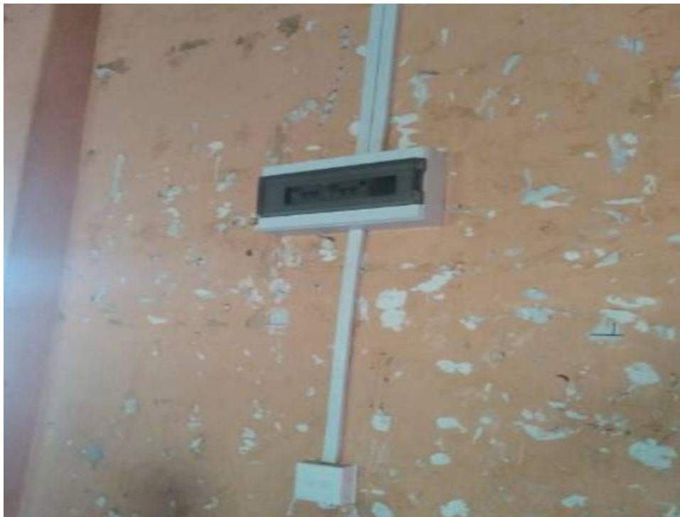
Figure 23 Electricity work at V/ Suntharapuram Sar
