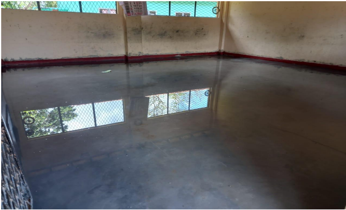
Figure 7 Repairs to class room Building at V/Puliyankulam Primary School
