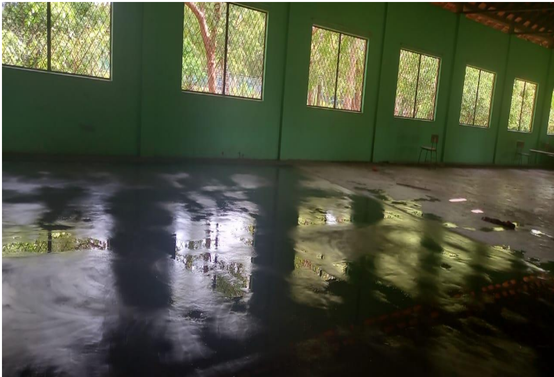
Figure 15 Repairs to class room Building at V/ Tharanikkulam Ganesh Vid
